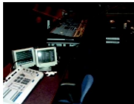
The lighting control for the house is achieved through an ETC Expression 3 console supplied by Paul Luntsford at PLA Designs.
